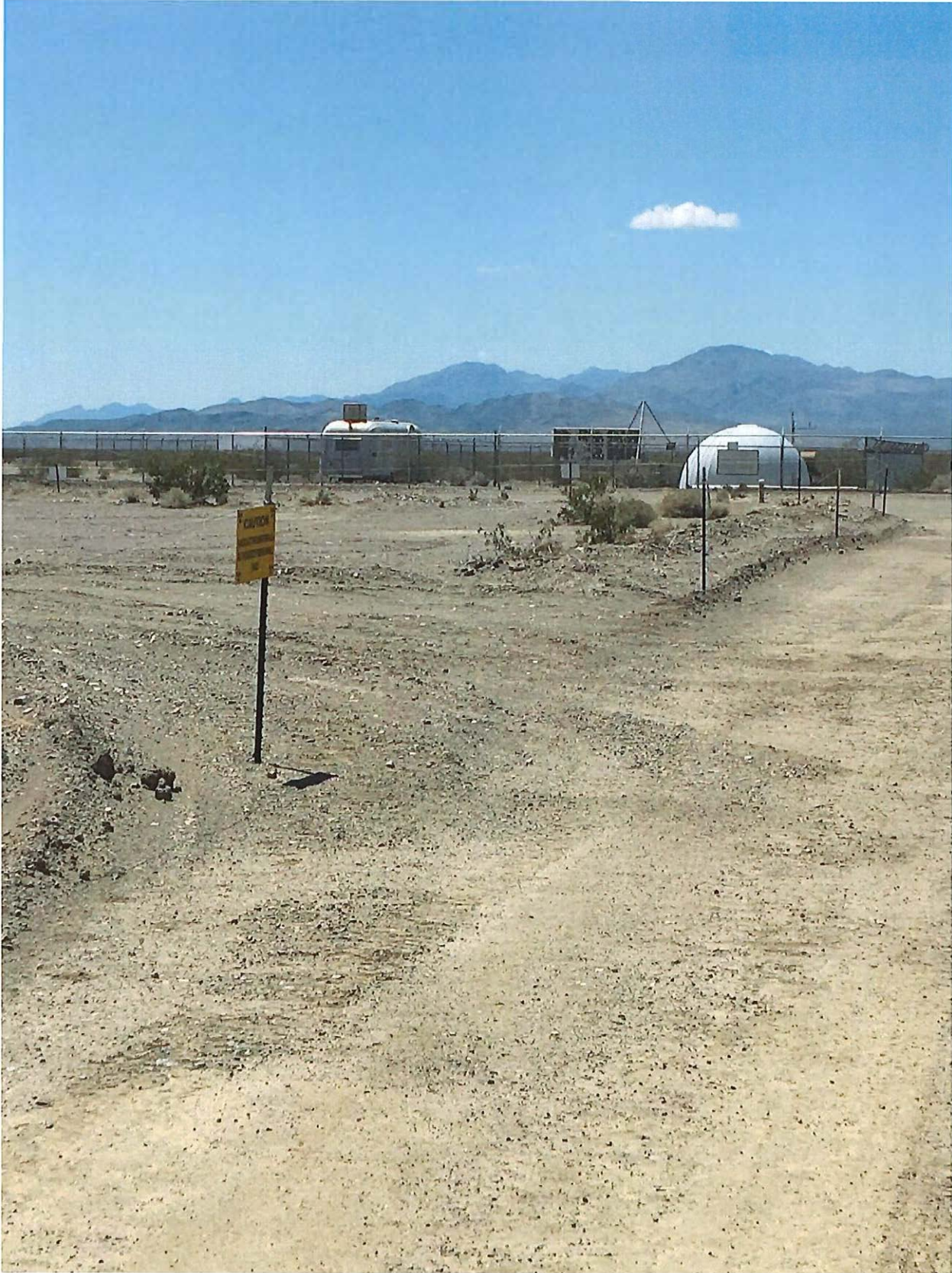
Interior Cap Boundary with Perimeter Fence
